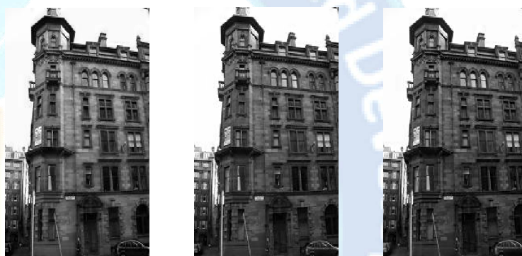
Fig 3(a) Gray level image of 'glasgow3.jpg' showing intensity in RGB planes (from left to right).
