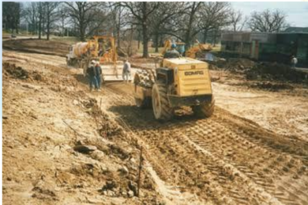
Fig. 1: An Image of Soil Stabilization Using Fly Ash
