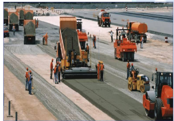
Fig. 2: Soil Cement Stabilization
